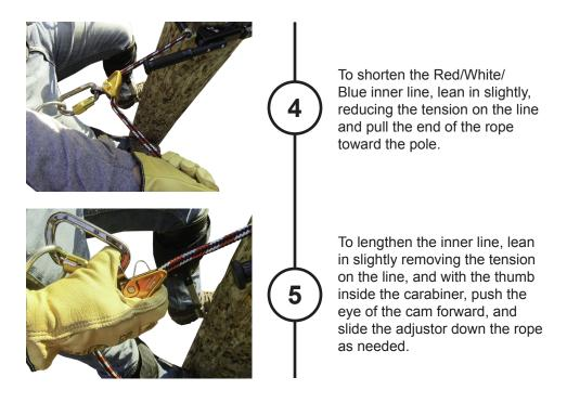
CAUTION! Remove your thumb from the cam before placing your weight back on the line.
